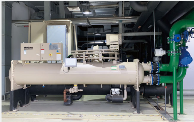
500RT inverter centrifugal chiller
